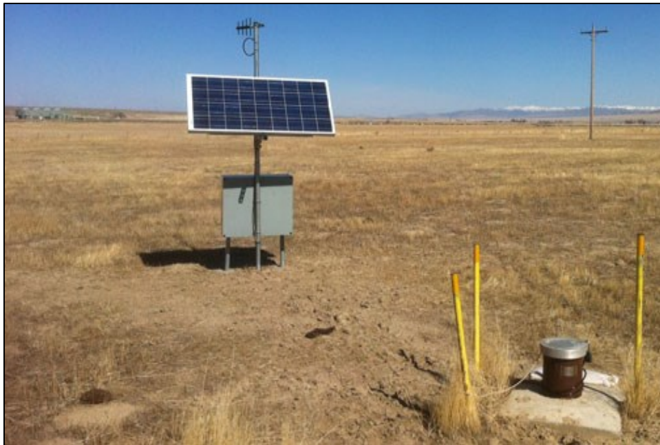
Figure 2-9. Surface equipment at a seismic monitoring site at the Raft River geothermal field.
